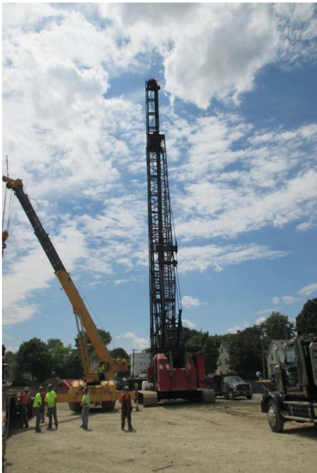
Installation of Foundations
