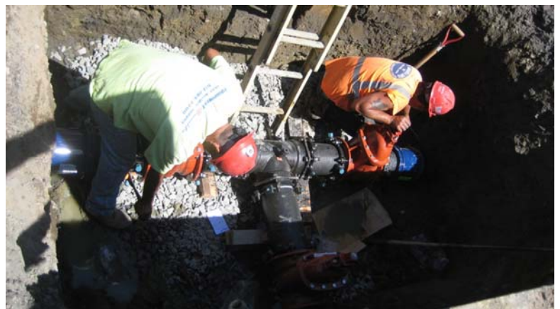
Utility Tie-Ins in Street
