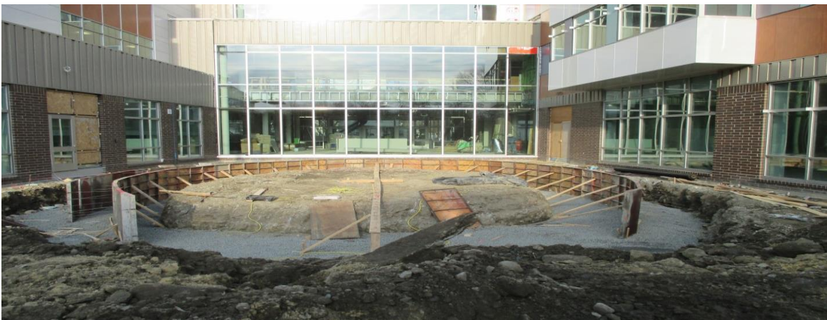
Status of Exterior/Interior Construction
