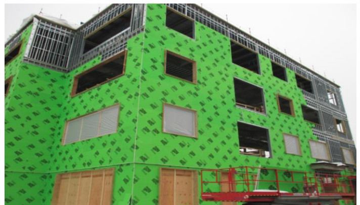
Interior Masonry and Exterior Wall Framing and Sheathing on TMMS
