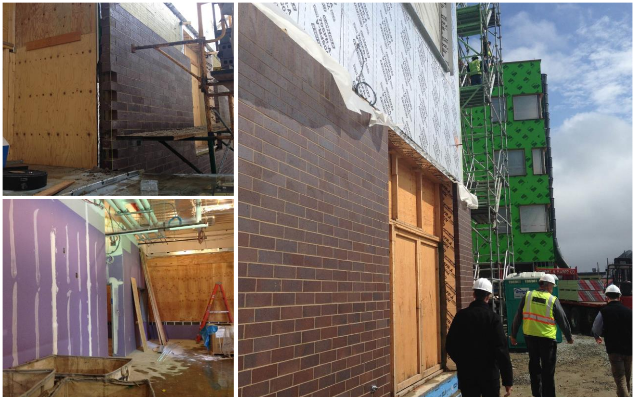
Status of Exterior and Interior Construction
