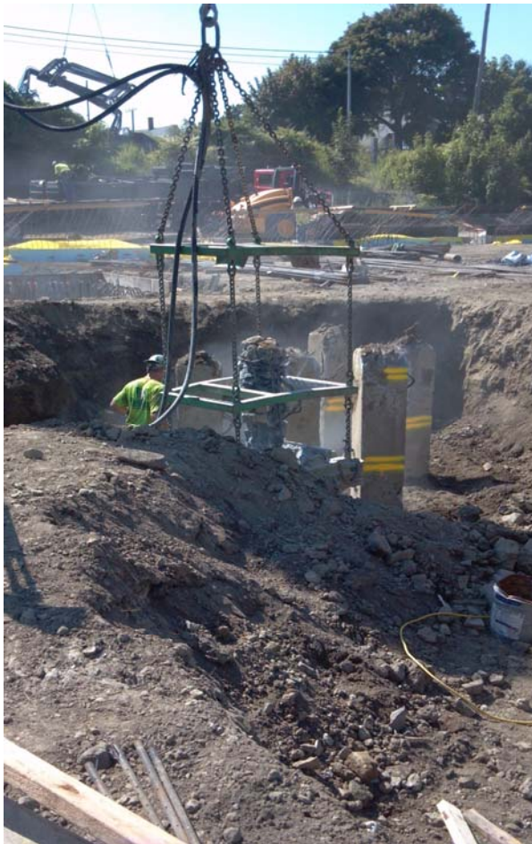
Cut-off Piles to Pile Cap Elevation
