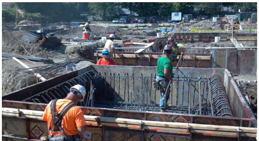
Installation of Pile Caps and Foundations
